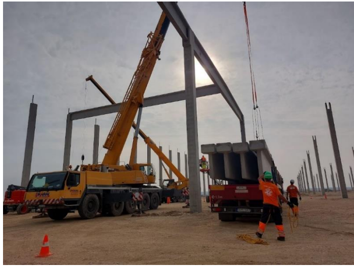
installation of the cross beam
