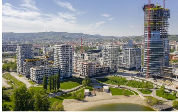
First years of BUDAPRT construction
