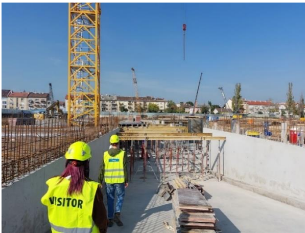
The construction site of Zugló
