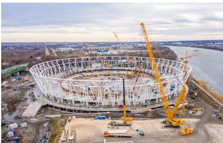
National Athletic centre – steel frame construction
